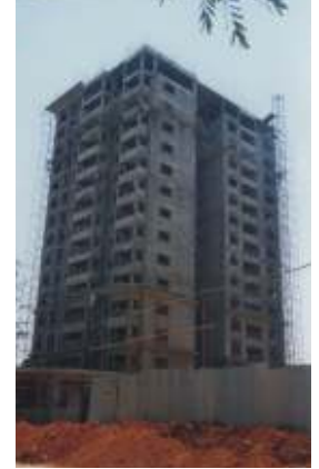
Magnolia Block construction nearing completion.
