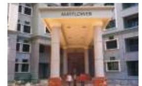
The entrance portico of the recently completed Mayflower Block.
