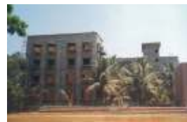
The school building nearing completion, as seen from the mini-stadium.
