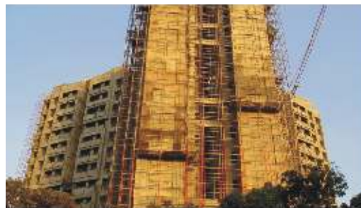
External cladding of Golden Magic Block in progress
